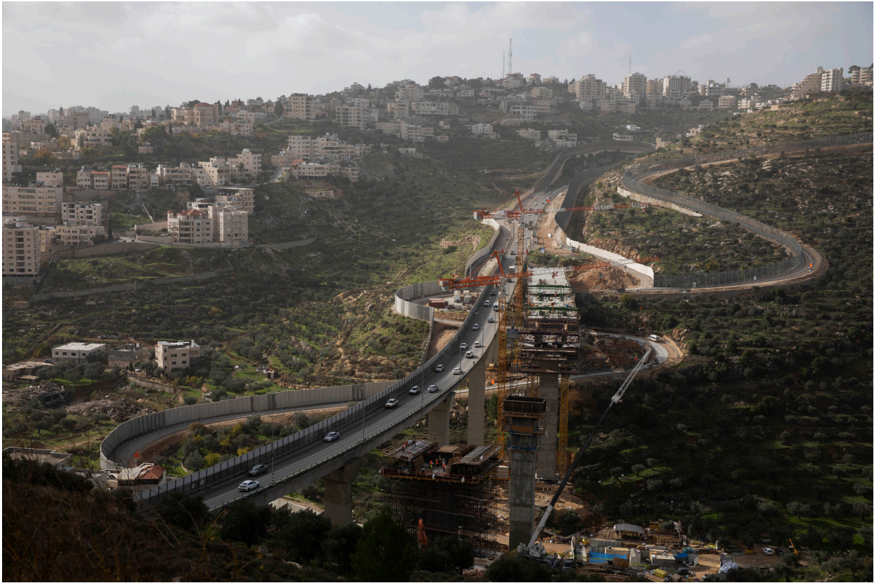
Tunnel Road (Route 60) | 15 December 2020 | Photo: Oren Ziv
