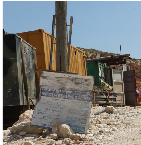
Bardala Bypass Pipeline construction site. Photo: Who Profits | 18.6.19
