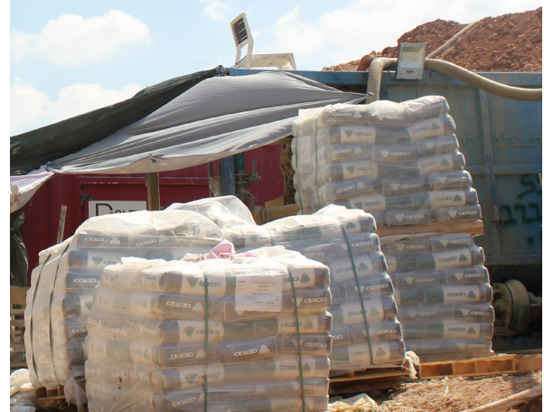
Bardala Bypass Pipeline construction site. Photo: Who Profits | 18.6.19
