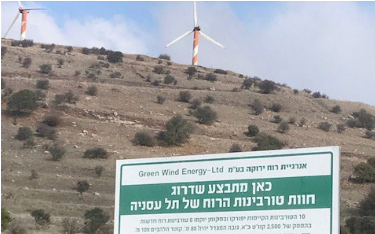
Project sign near Al-A'saniya wind farm, Occupied Syrian Golan. Photo: Who Profits. November 2018
