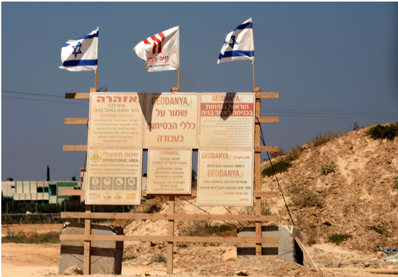
The entrance to the construction site of Danya Cebus. June 2018
